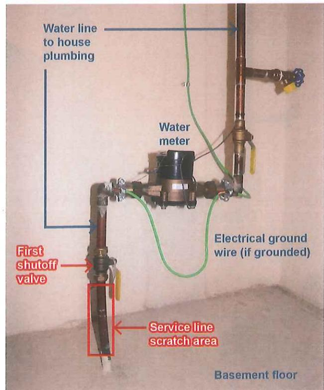
Scratch the pipe area coming into the house below the first shutoff valve. NOTE: The piping above the shutoff valve, known as the water line to house plumbing, should not be tested as it is likely made of a different material than the service line.
